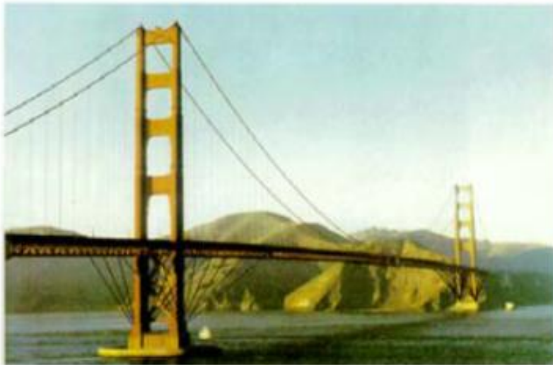
Double-sided Suspension Bridge
