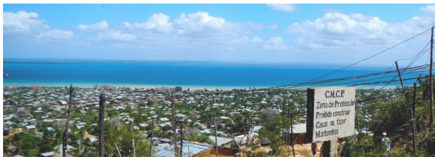
A sign reads “prohibited to build houses and farms” in a neighborhood in Pemba, where many landslides occurred in 2014. Several houses were destroyed and lives lost. Credit: Lécio Munguambe, CCAP/USAID
