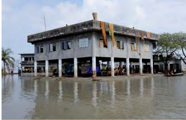
Figure 9.34 – A cyclone shelter in Bangladesh
