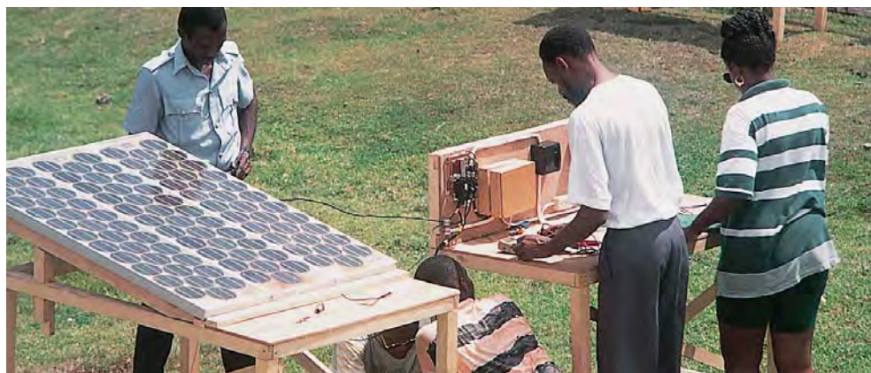
Figure 2.1 – Learning how to construct solar electric systems in Africa
